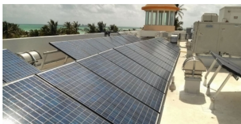
Florida Governor Extends Tax Exemption for Renewable Energy Installations
